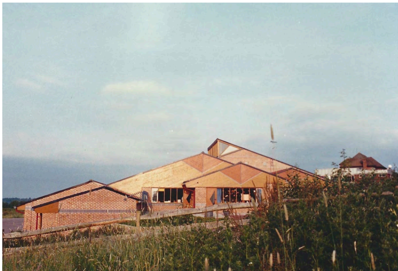
Battle Langton Primary School, 1986. A composite of classrooms clustered together across and down the hillside: section and elevation.
