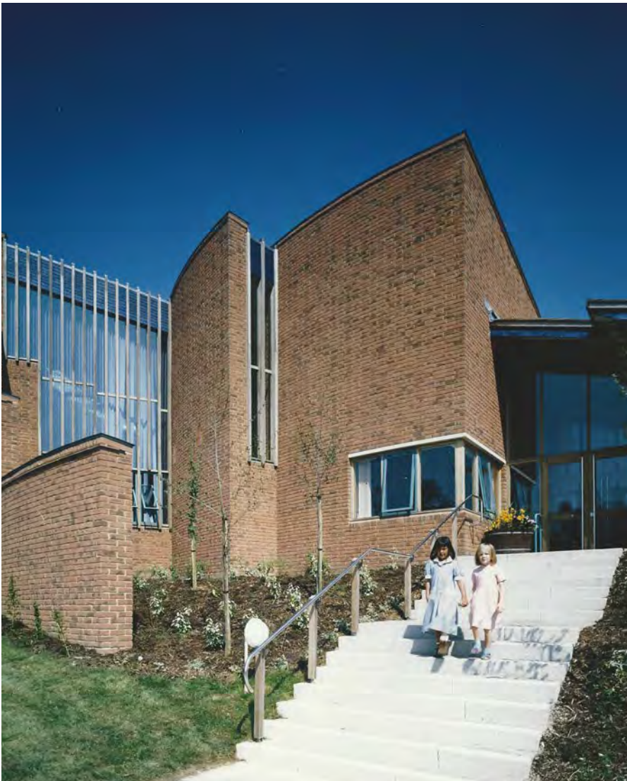
Solent Infants School: staff entrance with assembly hall on the left. The brick modelling and timber mullions were strongly influenced by Aalto.
