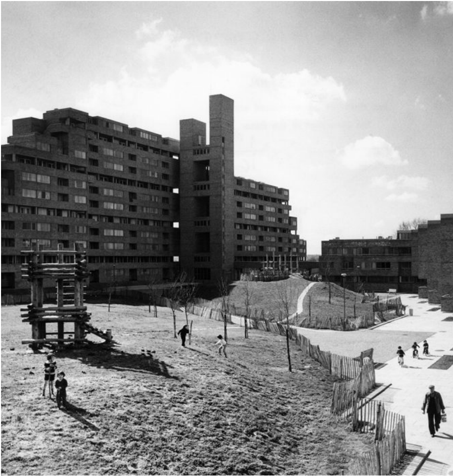
The scale of the central courtyard in Dawson's Heights instills a sense of enclosure and protection for residents, who, from their apartments have a view ten miles across London.
