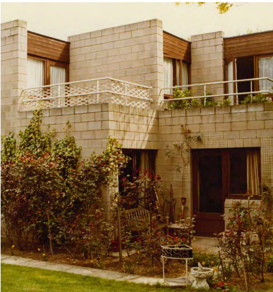
Macintosh Court: large format bricks make the massing more rugged in relation to the small scale of the blocks.
