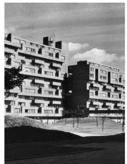
Dawson’s Heights, Southwark, London. Readable in the facade, split-level apartments are accessed from communal circulation balconies that occur every three floors.
