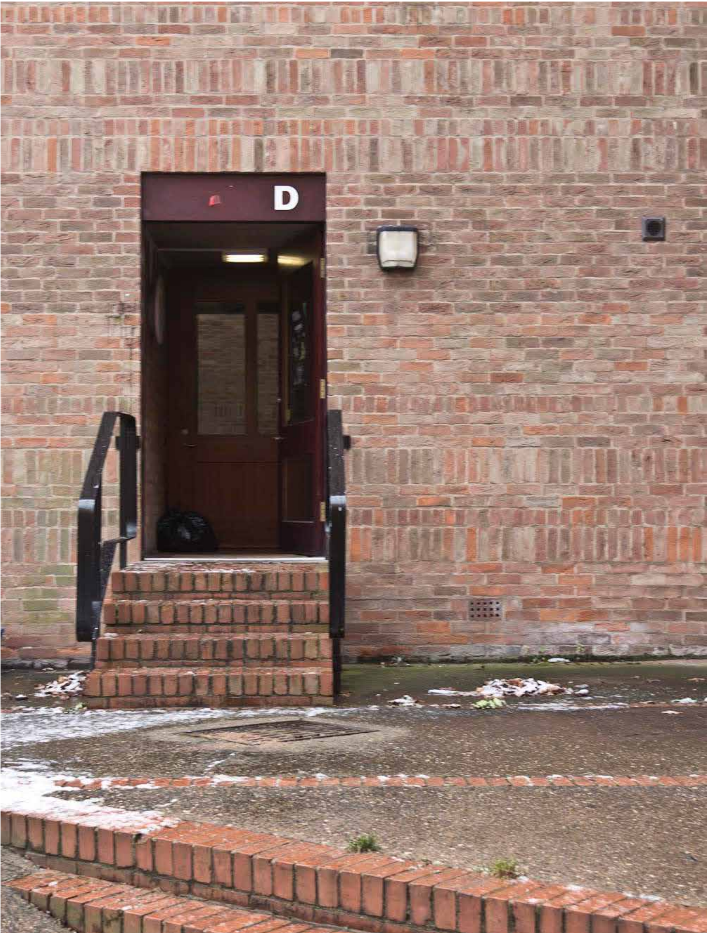
Entrance to the communal hall that leads to the student rooms.
