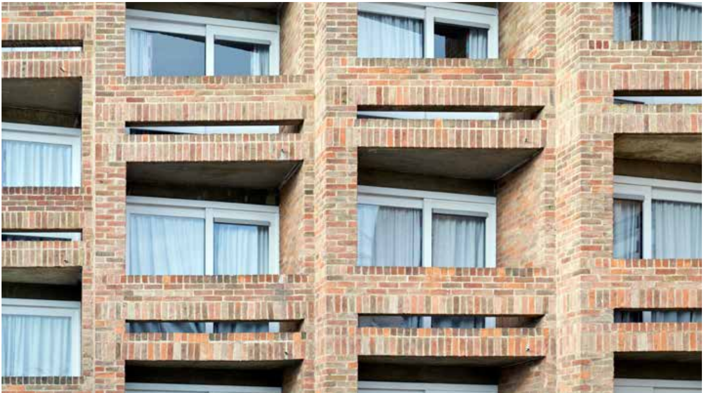
The horizontal lines in the facade brickwork are used for vertical fragmentation.
