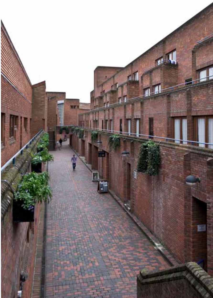
The walls of the inner street in which the galleries provide access to the student rooms. The street functions as a collective domain.
