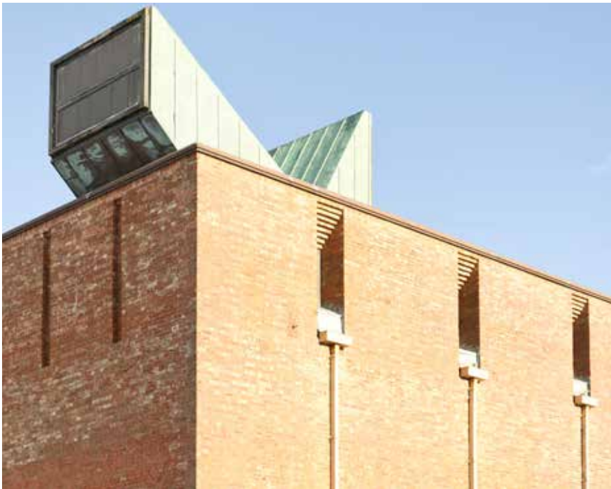
The northern end wall with 'tree patterns' as accents in the brickwork.
