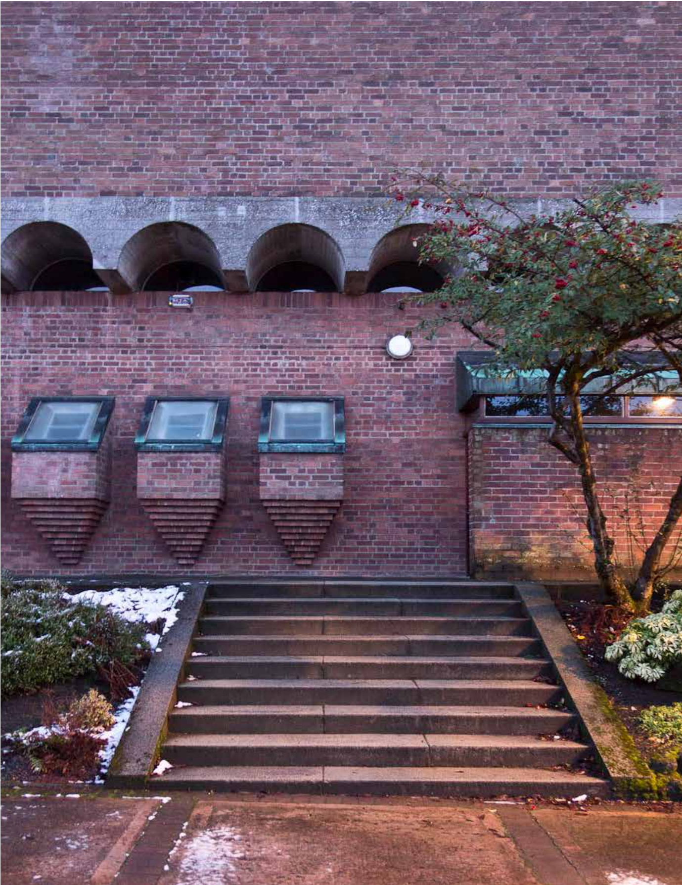
Fragment of the facade ornamentation that allows varying amounts of daylight to enter.
