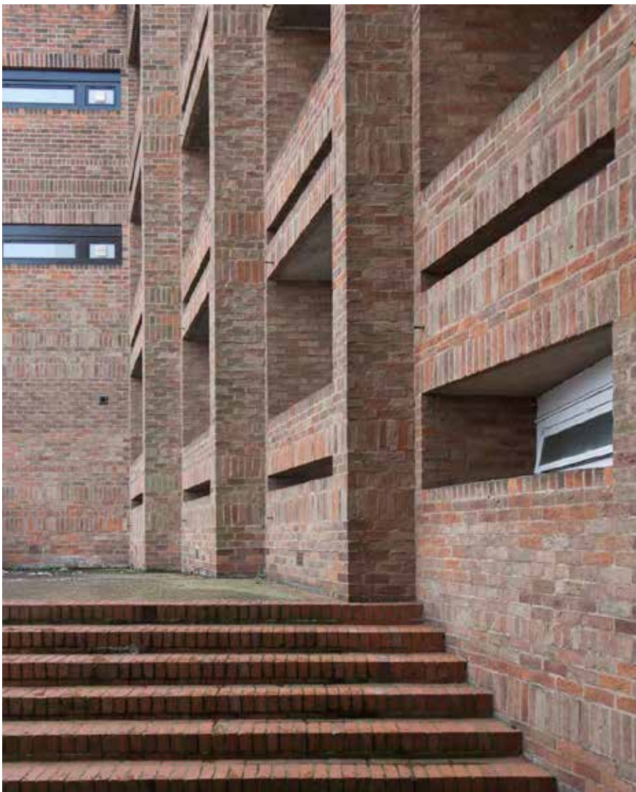
The horizontal lines in the facade brickwork are used for vertical fragmentation.
