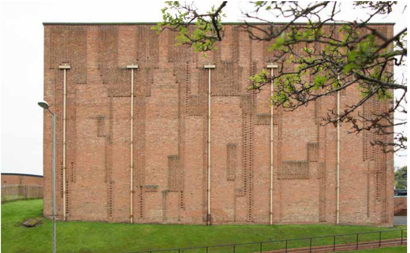
The northern end wall with 'tree patterns' as accents in the brickwork.
