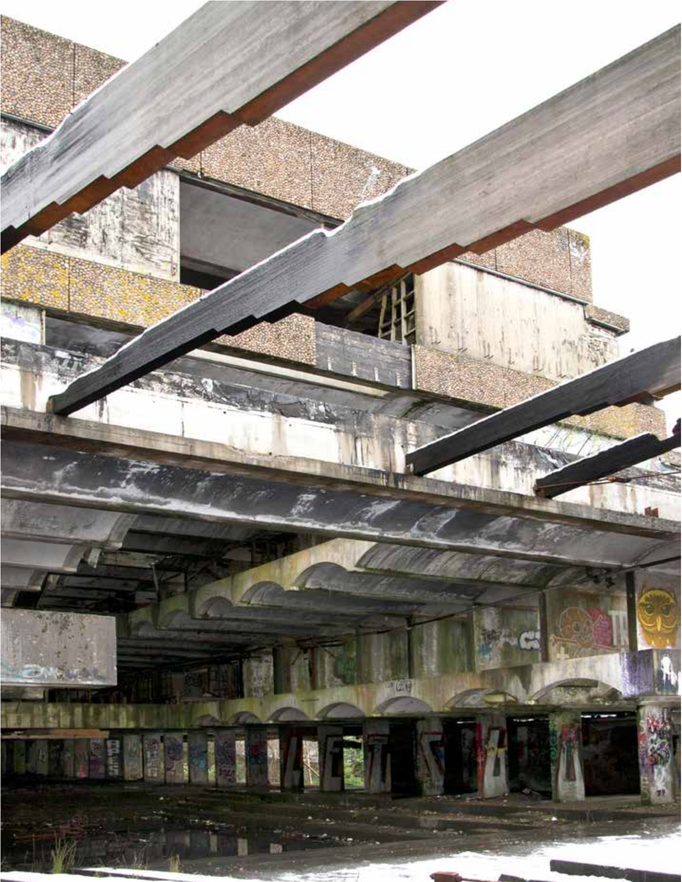
End of the main block, standing on the altar in the chapel, with the laminated beams still visible.
