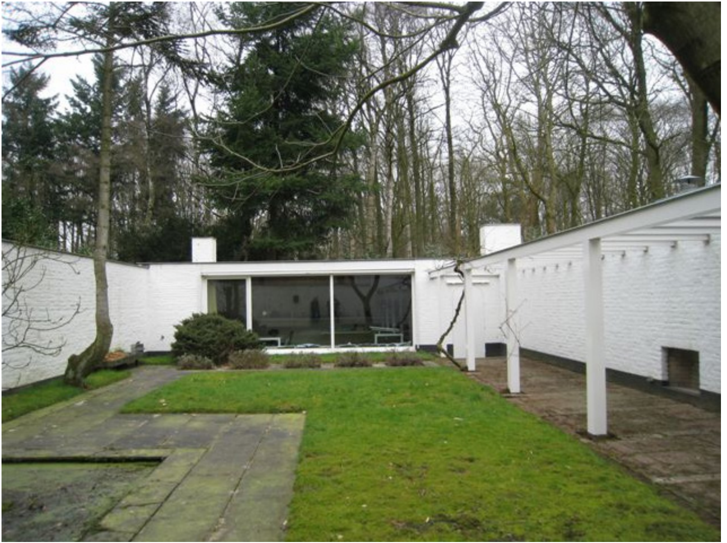
Private House Bedaux 1937, 1950 and Privékantoor 1960, Goirle
